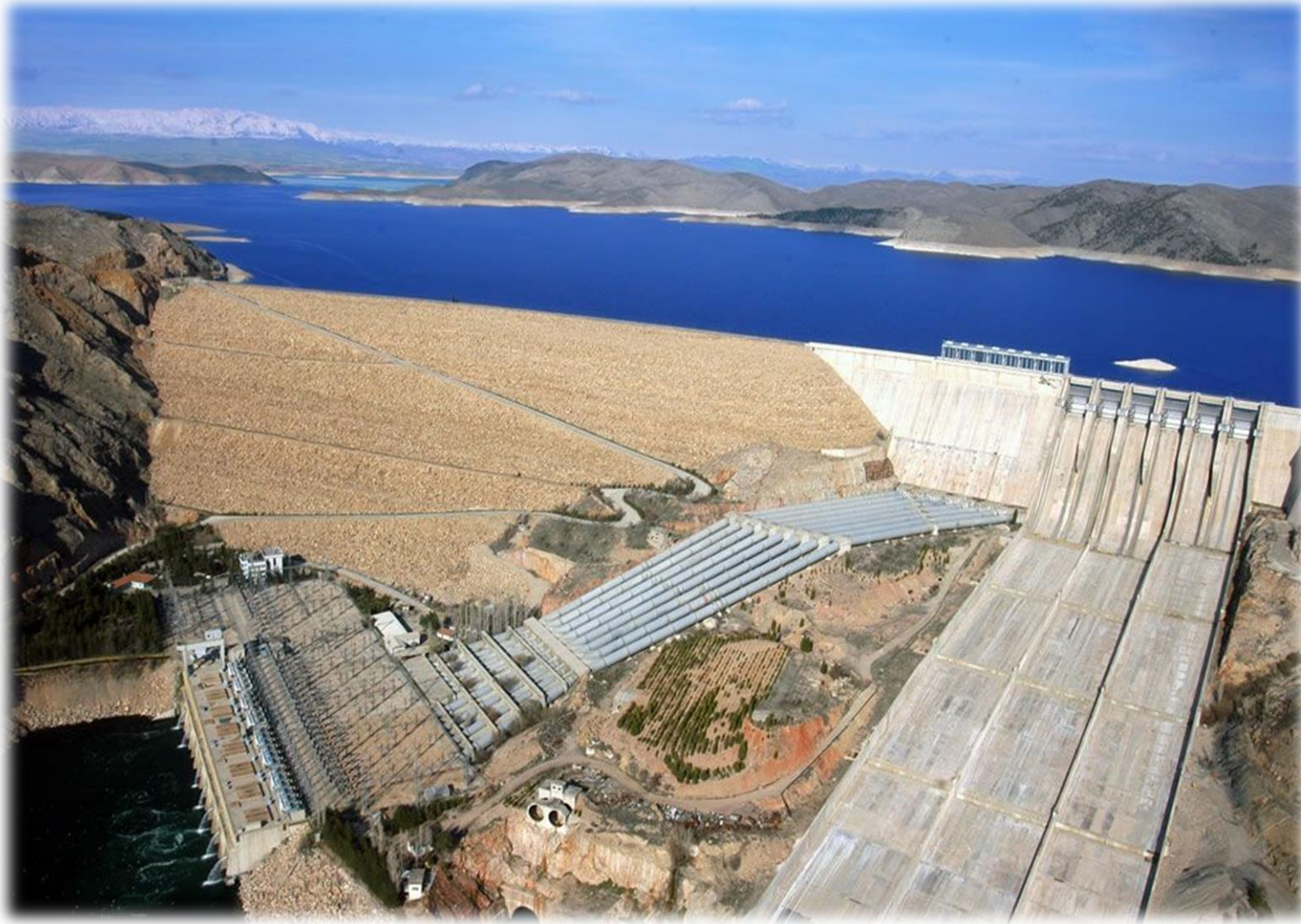
Keban Barajı, Elazığ
